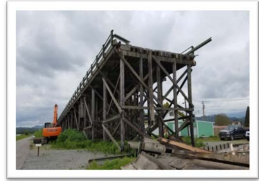
Demolition of the Burlington Northern Overpass (Old Hwy 99)
