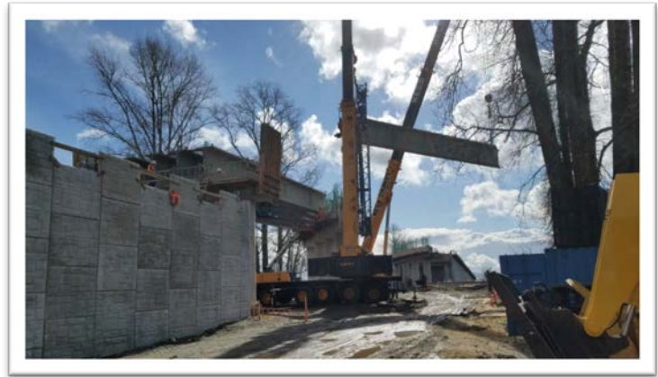
Construction of the new Burlington Northern Overpass
