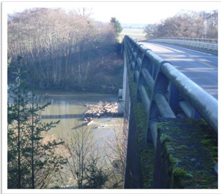
Debris on the North Fork Bridge
