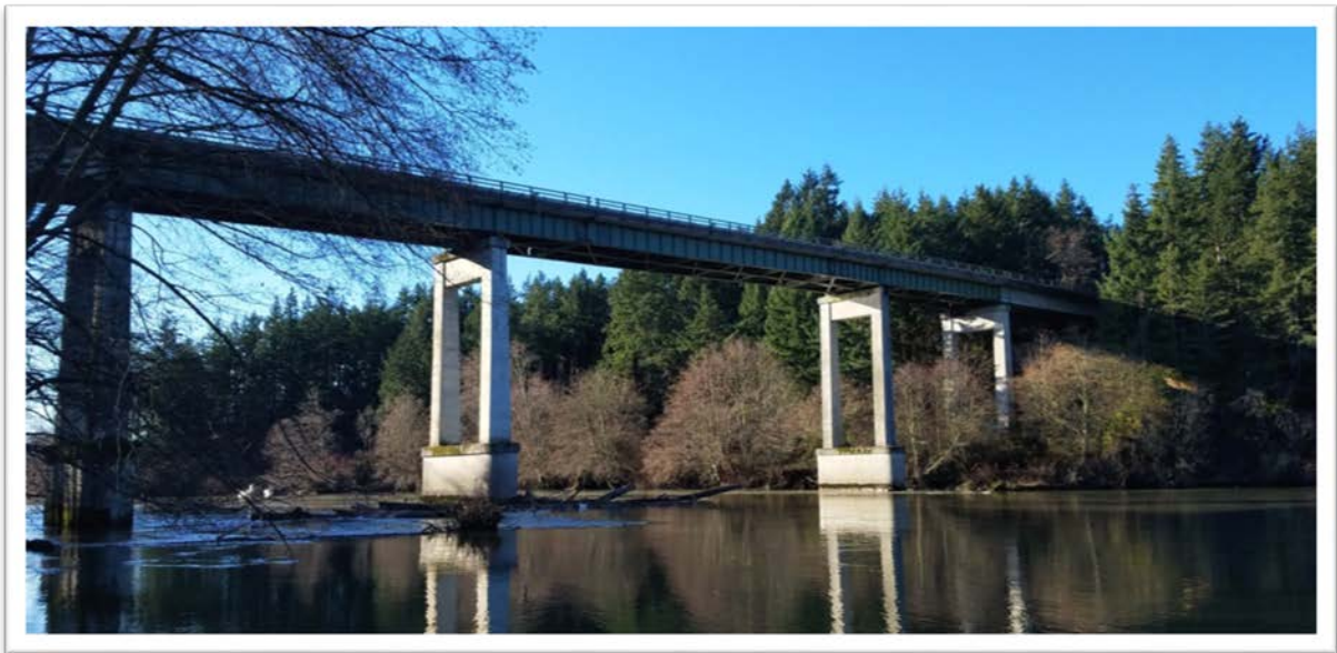
North Fork Bridge (Best Road)
