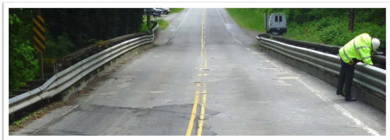
Friday Creek Bridge on Old Highway 99 N, deck covered in concrete patch repairs.
