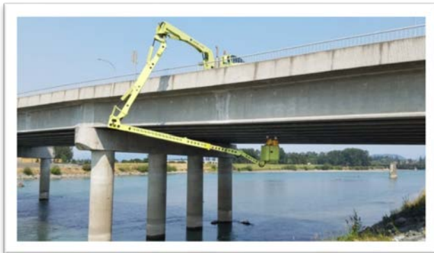
UBIT inspection on Riverside Bridge (City of Mount Vernon)
