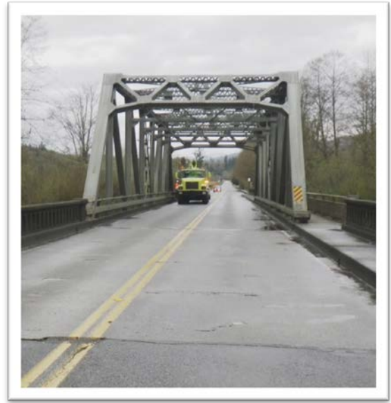
Samish River Bridge deck during inspection
