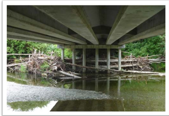
Debris under S. Skagit Hwy at Day Creek
