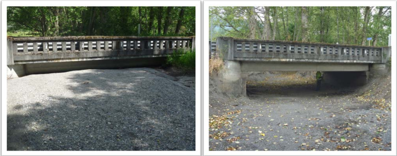
Before and after of Lyman Hamilton Highway at Childs Creek
